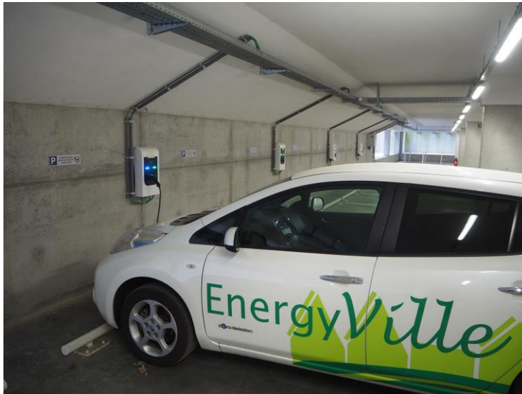
Figure 24 -EnergyVille office building: EV charging equipment
