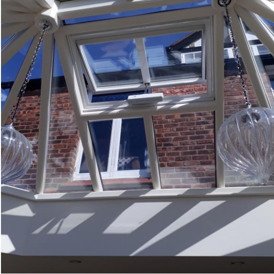
Figure 20 -Automatic smart conservatory top vent
