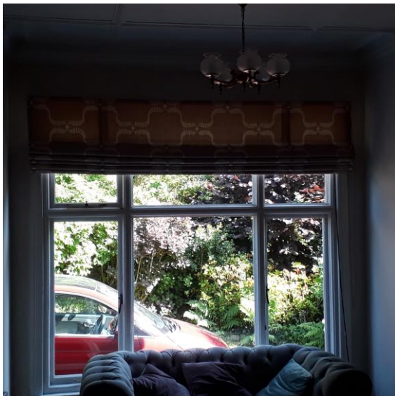
Figure 20 -Manual blinds/shutters for solar control and thermal comfort
