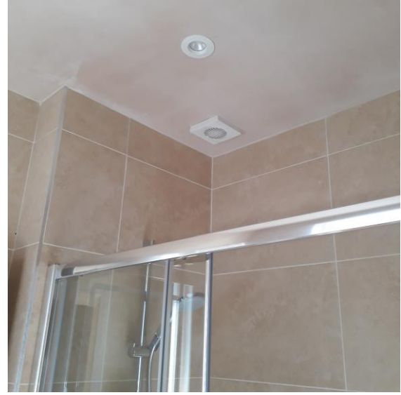
Figure 19 -Ventilation only via extractor fans
