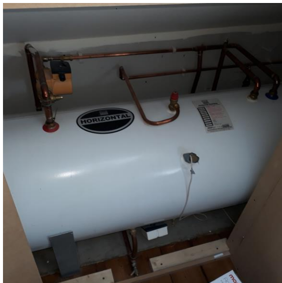
Figure 24 -System boiler and hot water storage tank
