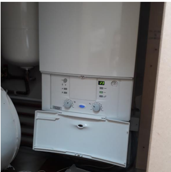
Figure 24 -System boiler and hot water storage tank
