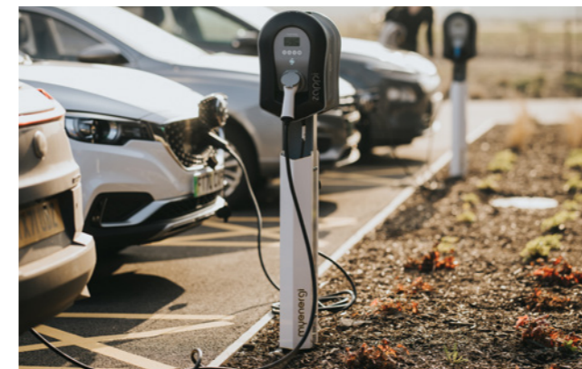
Some chargers come with a built-in RFID reader to allow controlled activation of charging, for both private and workplace use. Note that the RFID card is used to initiate charge (not for payment functionality).
