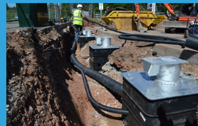
Civils infrastructure being installed
