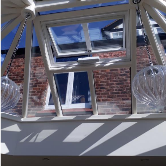
Figure 37 - Automatic smart conservatory top vent
