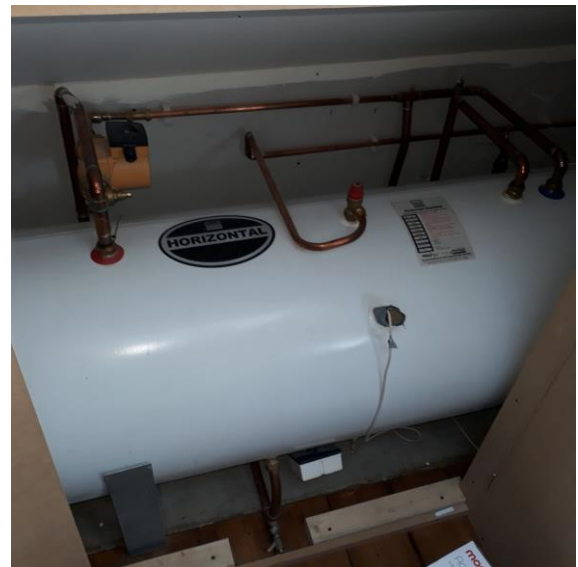
Figure 41 - System boiler and hot water storage tank
