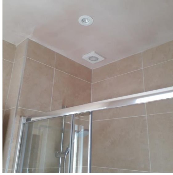
Figure 35 -Ventilation only via extractor fans
