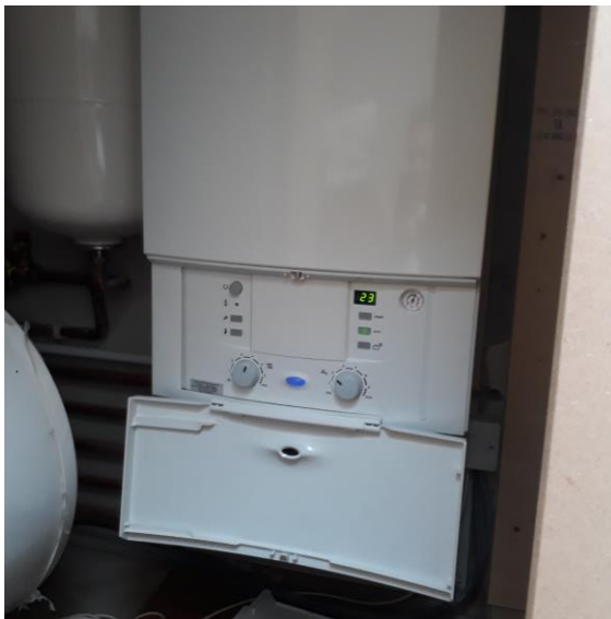
Figure 41 - System boiler and hot water storage tank
