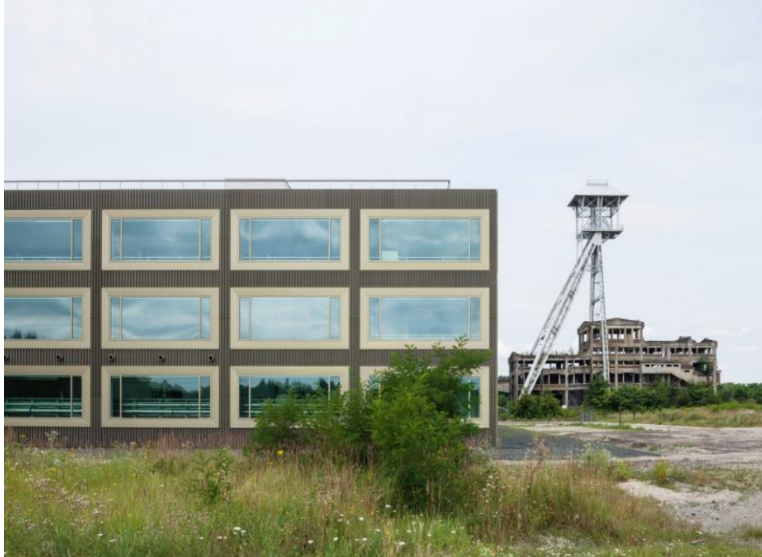
Figure 45 -EnergyVille office building assessed in field study - rear view
