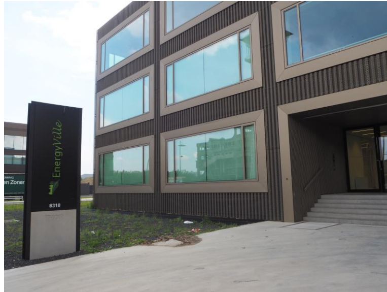
Figure 43 -EnergyVille office building assessed in field study – front view
